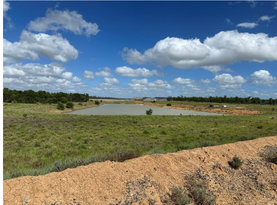
Photo 14: Southern Sediment Dam (10 December 2025)
