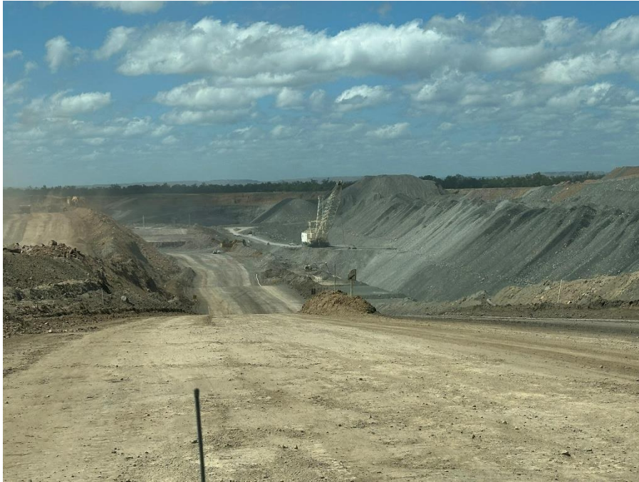
Photo 19: Pit with dragger Dragline (10 December 2025)
