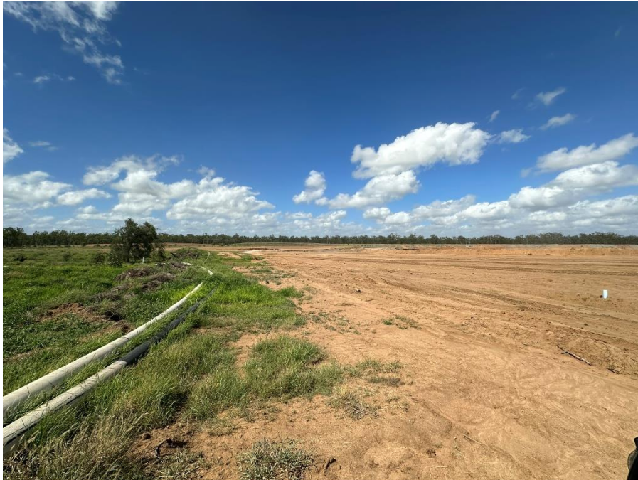
Photo 15: Isaac Downs Highwall (Southern End) - recently topsoil stripped. (10 December 2025)
